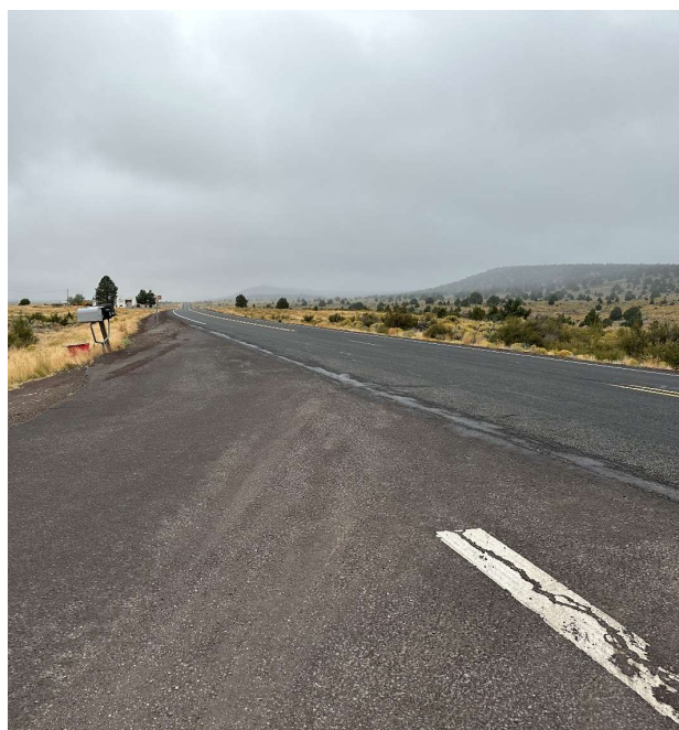
Figure 2. Pine Mountain Road Facing West
