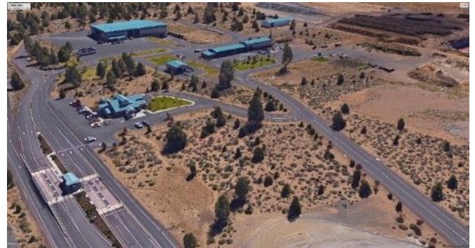
Knott Landfill Recycling and Transfer Facility is located in Deschutes County just outside the southeast corner of Bend city limits.
