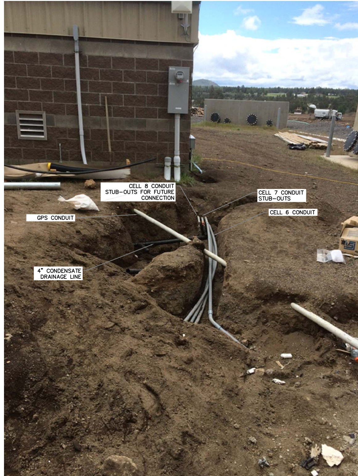
A EXISTING CONDUIT STUB-OUTS M6
