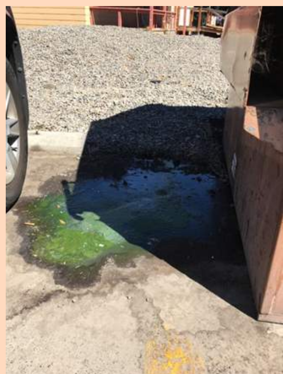
Photo 2. Sewage overflow in public parking lot
