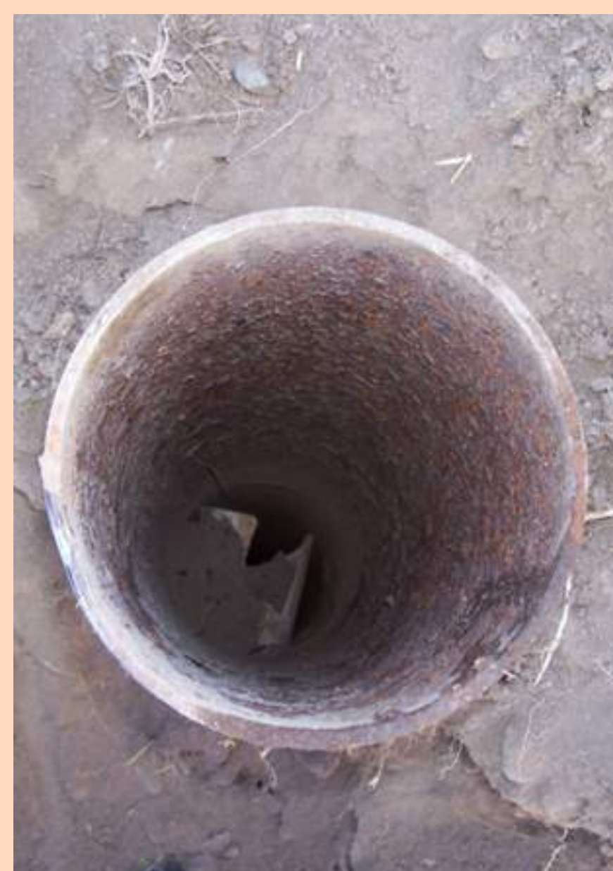
Photo 3. Drillhole injecting effluent into the ground
